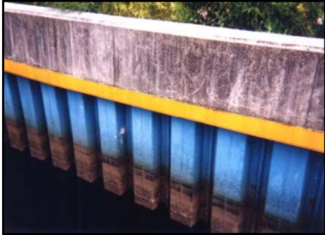
Steel Sheet Piling
