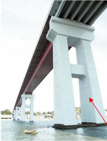
Wrap-around reinforcement of Reinforced Concrete Bridge Support
