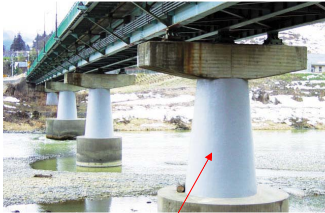
Wrap-around reinforcement of Reinforced Concrete Bridge Support
