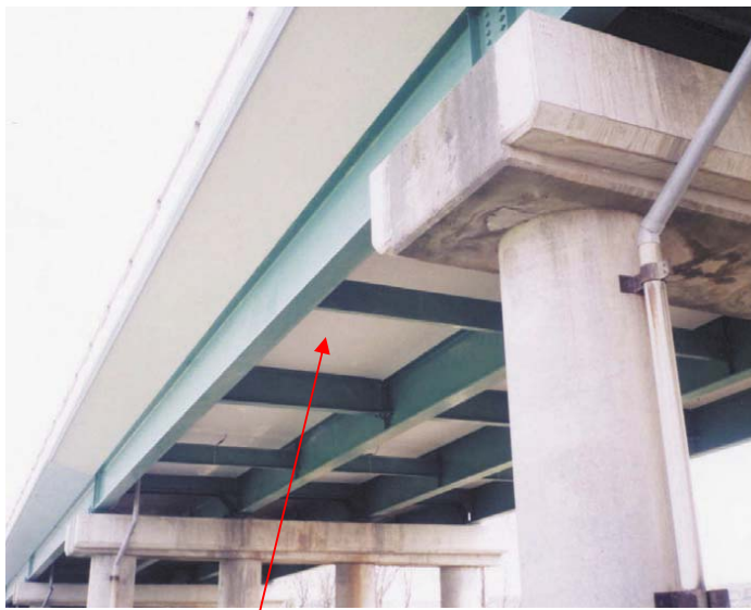
Lower Surface Reinforcement of Reinforced Concrete Floor
